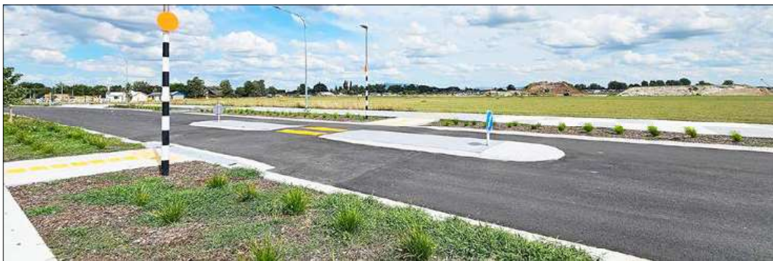
Ready to go: Bus and turning bays, footpaths, landscaping and crossings are all in place ready for the school opening.
